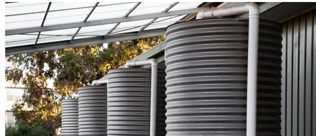
Precipitation is expected to become more unpredictable due to climate change, with periods of excessive rainfall (causing flooding) and very limited rainfall (causing droughts). Rainwater storage can hold excess rainfall to be used when rainfall is limited.
