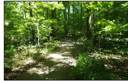
Figure 16: Improved trail surface
